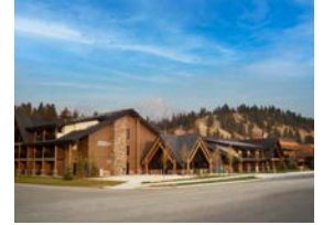
Forest Park Hotel NEW - Ongoing renovation
